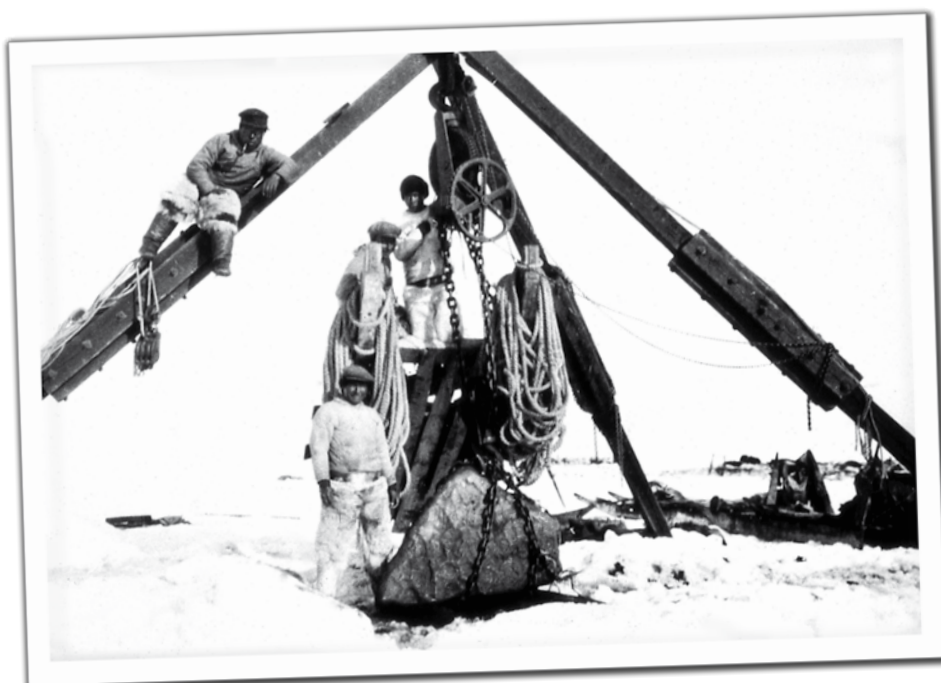
Figure 1. The iron meteorite Savik is hoisted up from the ground. Today it sits in the yard of the Geological Museum. ©V.F. Buchwald.
